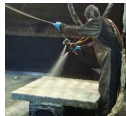
Polyurea application process
